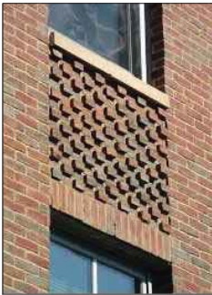
SAMPLE IMAGE PROJECTING BRICK DETAIL PANELS
